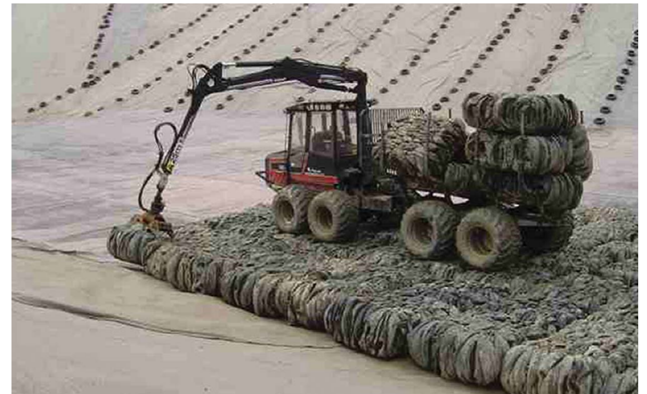
Figure D.14 – Tyre bales being placed in a leachate drainage layer at the base of a landfill cell at Bryn Posteg
