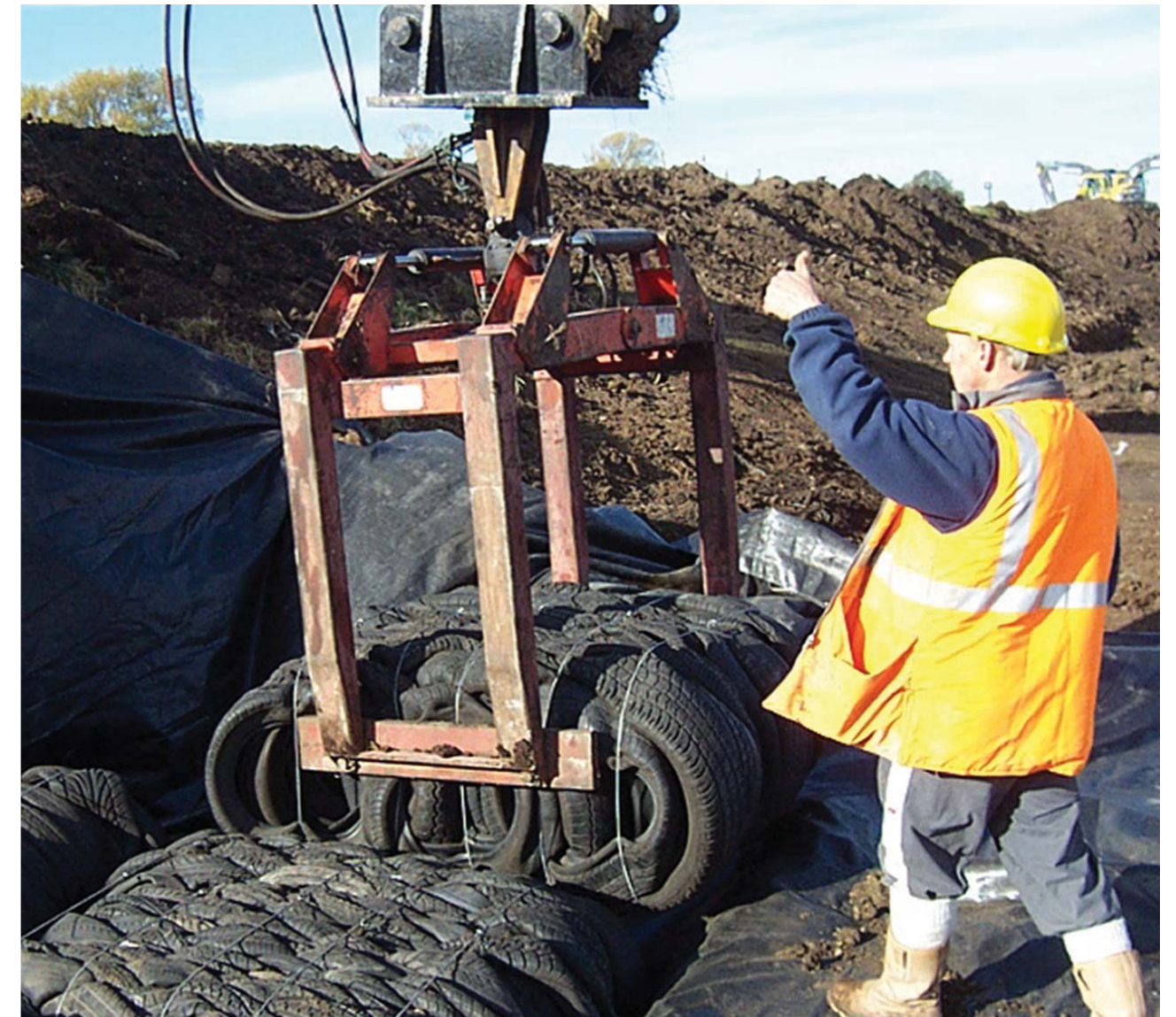
Figure D.5 – Placing tyre bales (using a pallet grab) within a wrapping of geosynthetic
