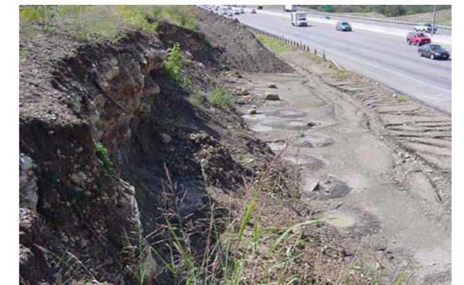
Figure D.8 – Excavated slide failure
