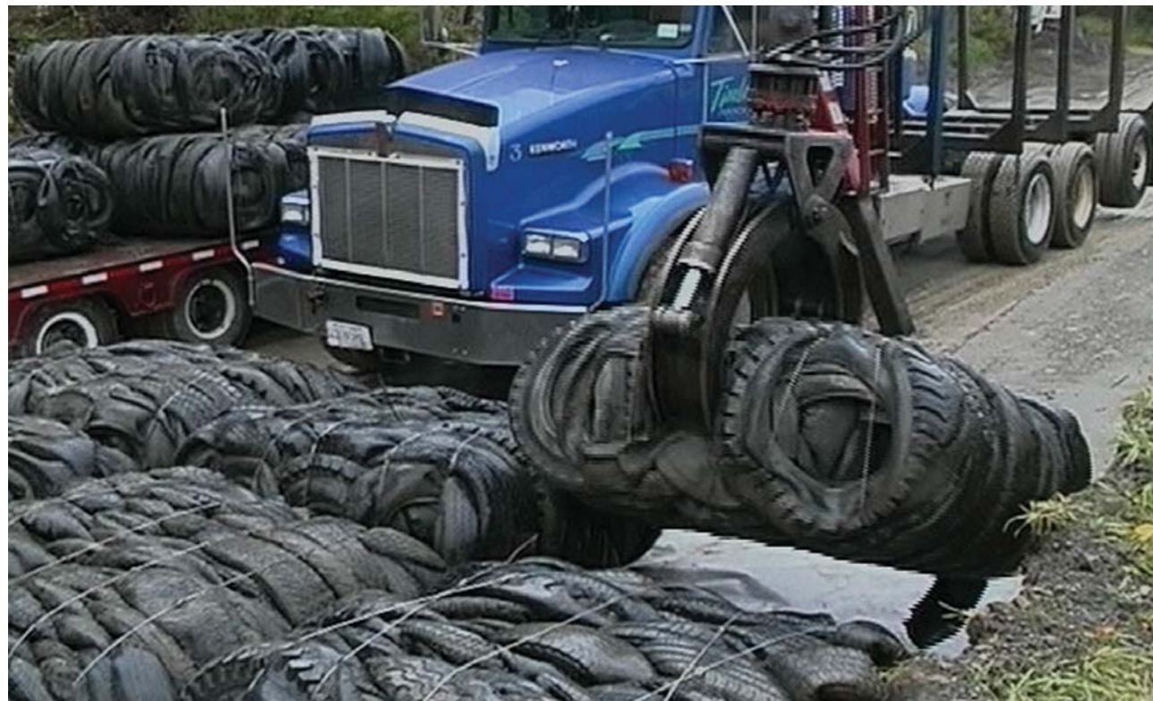
Figure 14 – Placing tyre bales using a ‘loggers’-clam’
